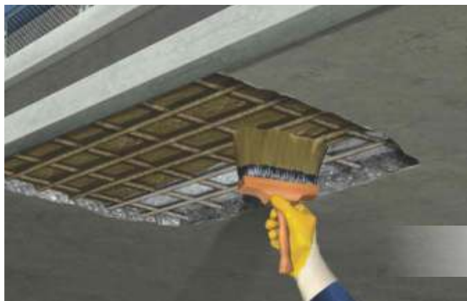
Anti –corrosive / Epoxy Coating of Reinforcement in RC
