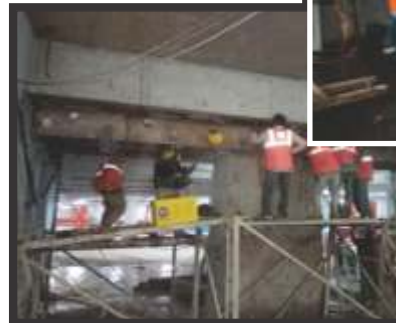
Tunnel strengthening with steel fabrication - Leela Palace.
