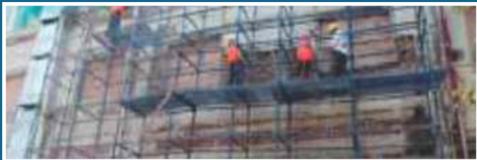
Removing Existing Plaster
