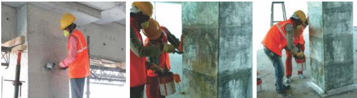
Glass Fibre Wrapping – KCT, Bangalore
