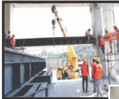
Structural beam fixation - KCT Site, Bangalore
