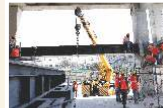
Structural Strengthening Fabrication
