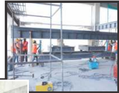
HEM Section 600 Erection Work - KCT, Bangalore
