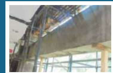
Finishing existing Beam with micro concrete
