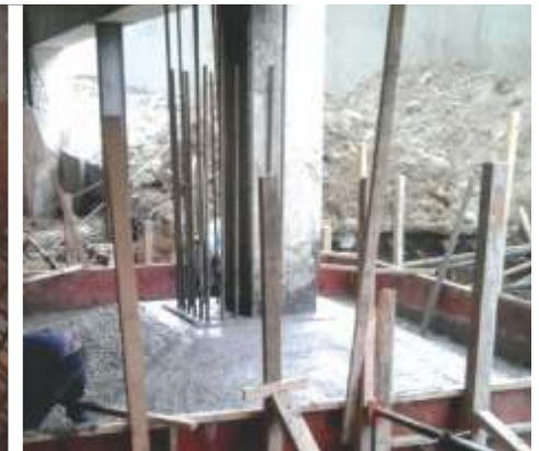
Strengthening of Foundation
