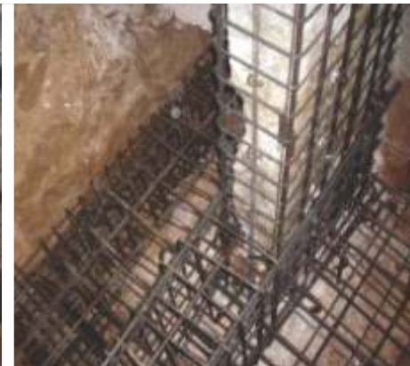
Strengthening of Foundation
