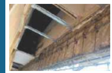
Reinforcement work with Shear Connectors
