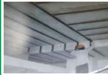
Carbon Laminate – 50/100mm wide – Tulip Data Center, Bangalore
