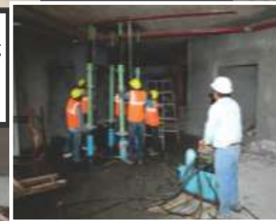
Slab uplifting and plate fixing, - KCT.
