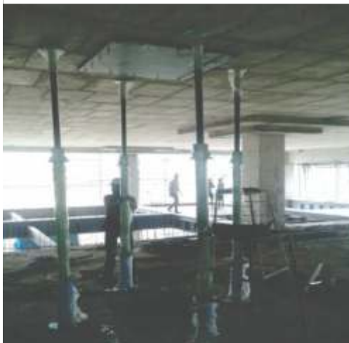
Up Lifting Existing Slab by Hydraulic Shafts – Tulip Data Center, Bangalore
