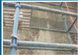
Applying 2.5 mm Weld Mesh
