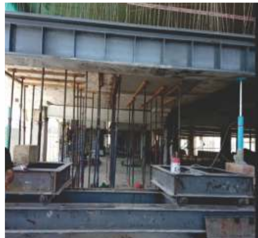
Elevating ISMB 600 Section steel double girder – KCT, Bangalore
