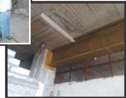
Structural Steel Strengthening, ISMB 900 - Mantri, Jupiter
