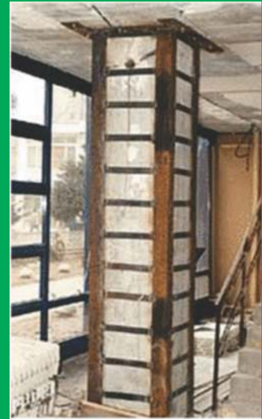
Steel Stirrup Jacketing – Net Magic Data Center, Mumbai
