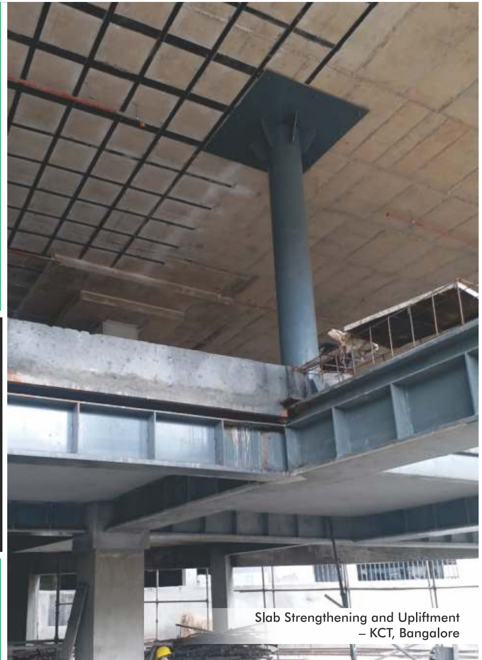
Elevating ISMB 600 Section steel double girder – KCT, Bangalore
