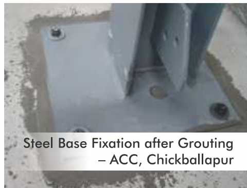
Epoxy Grouting – AMR Tech Park, Bangalore
